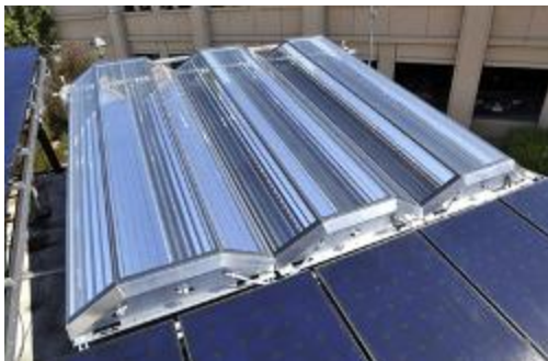
Figure 2: MCT systems installed as part of a domestic rooftop solar power system.
