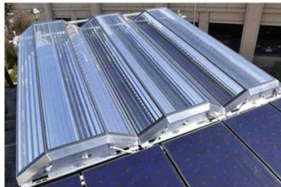
Figure 4. Micro-concentrator system on Santa Clara University Solar Decathlon House, 2010. The three MCT units were mounted on the same PV supports vacated by previously installed PV panels.
