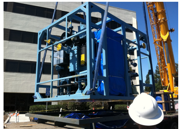
Lifting the Thermax absorption chiller to the CCMC roof
