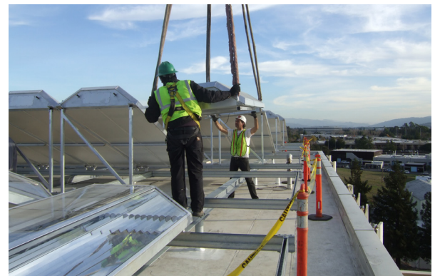
All 75 Chromasun MCTs were lifted and set in a single day
